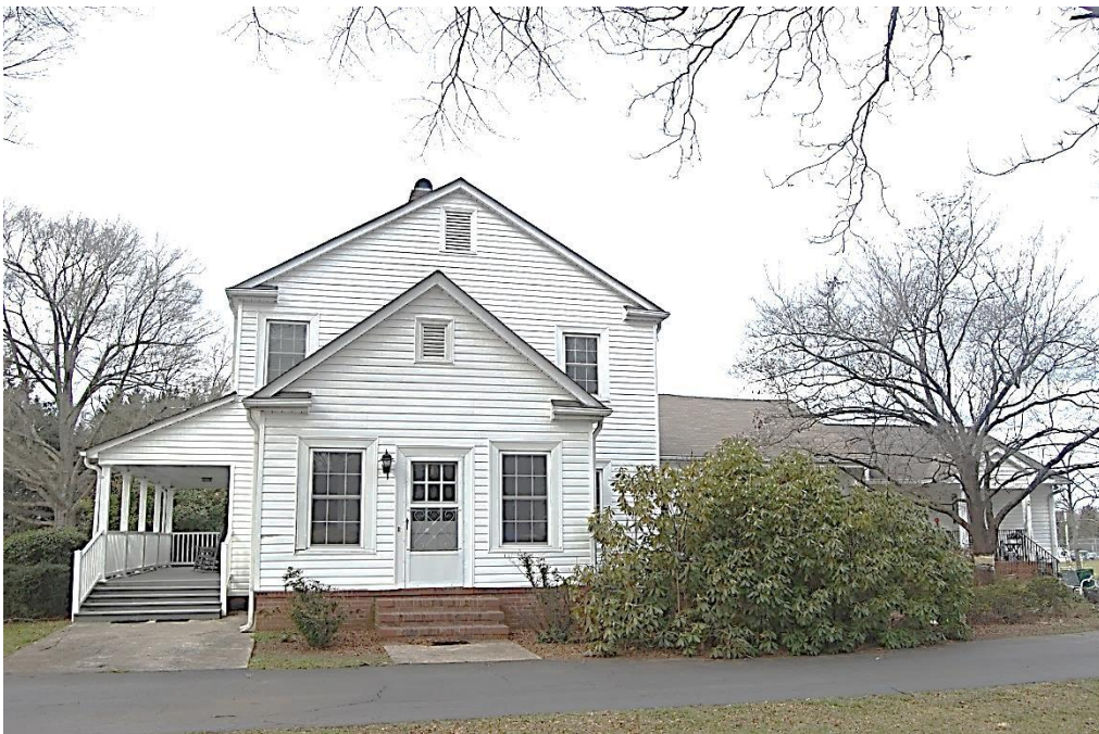
Hugh M. and Louisa C. McAuley House, Side (East) Elevation, Looking West.
