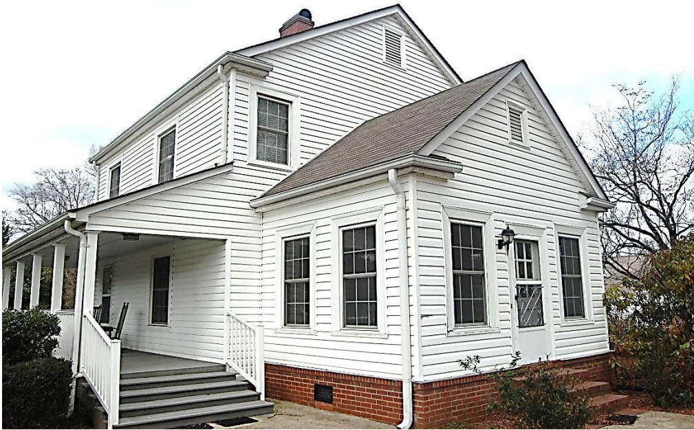
McAuley House, Façade and East Elevation, Looking Northwest.
