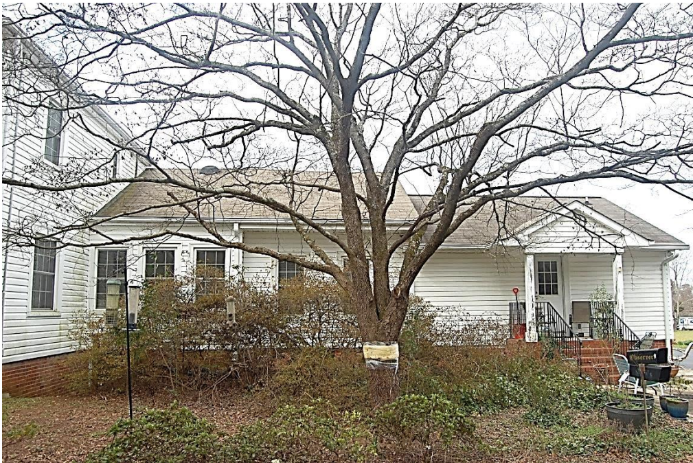
Hugh M. and Louisa C. McAuley House, Rear Ell, East Elevation, and Garage Addition, Looking West.
