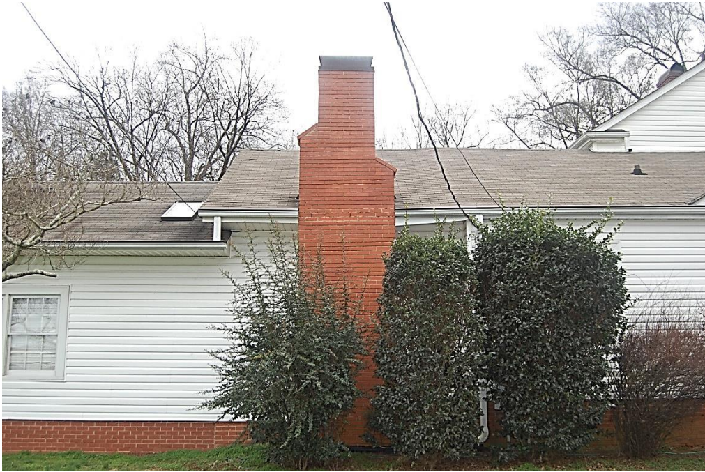
Hugh M. and Louisa C. McAuley House, Rear Ell, West Elevation, Looking East.
