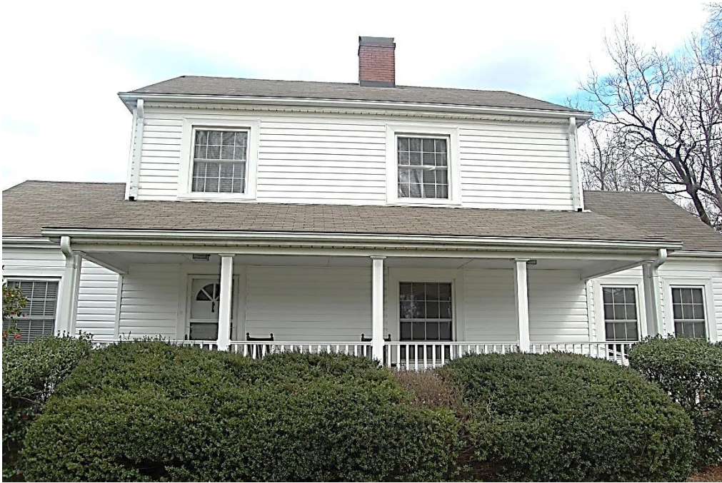
Hugh M. and Louisa C. McAuley House, Façade (South Elevation), Looking North.
